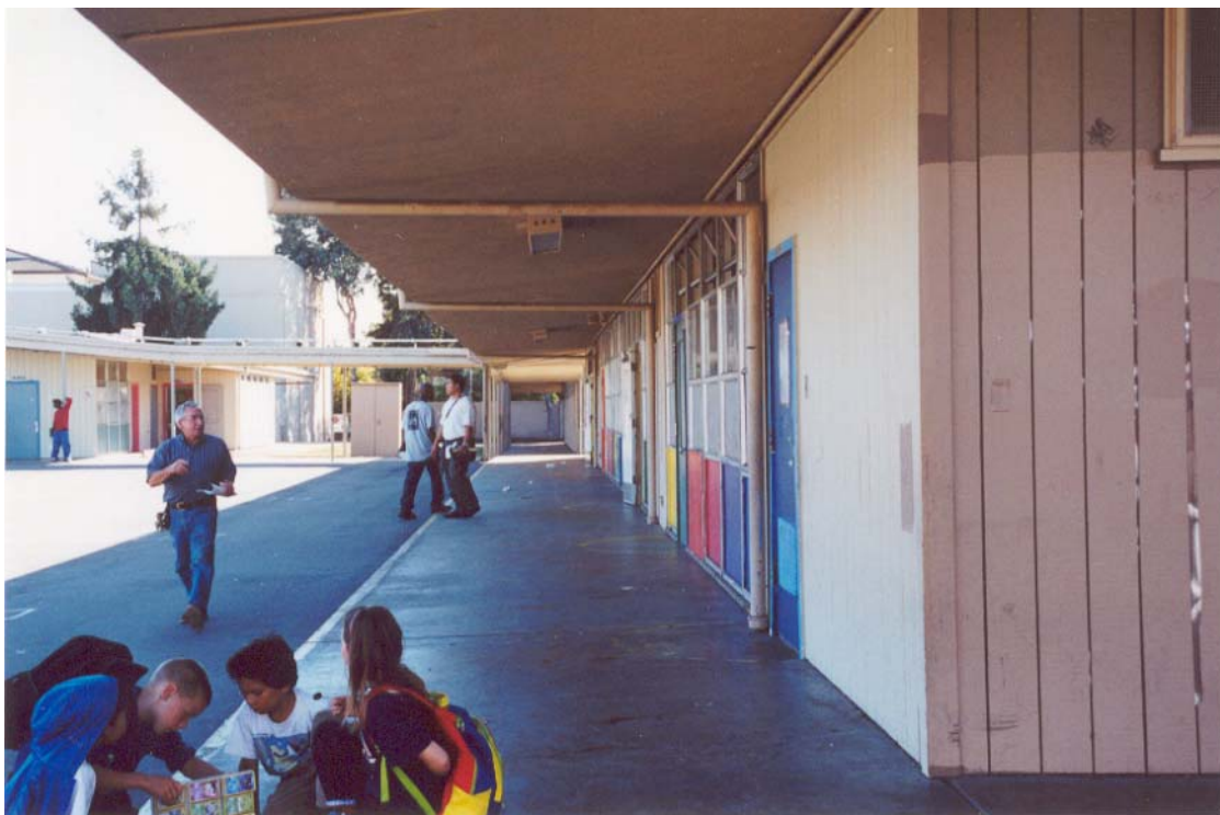
Figure 9: Covered Walkway Connecting Buildings.
