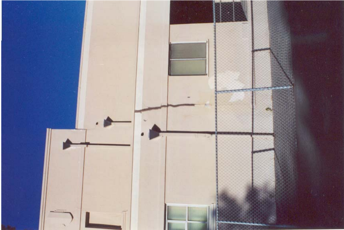
Figure 8: Multi-Purpose Building – Cracks in Plaster.
